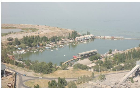
Figure 13. Andreev Bay, 1990s. An old trestle for loading grain from railway wagons onto ships can be seen
